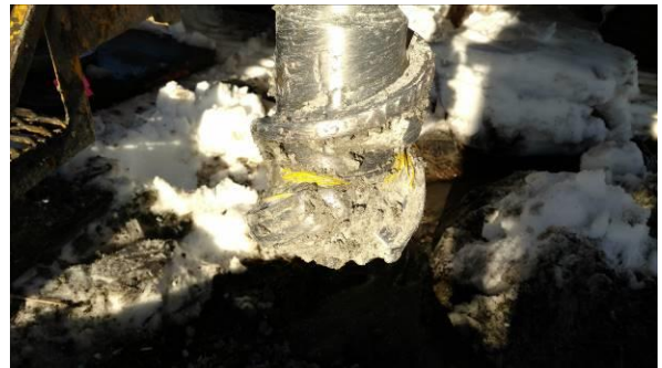
Photo #10 View of wiring wrapped around the auger from borehole 1358-9 (3).
