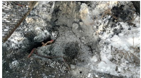
Photo #12 Sealing completion of borehole 1358-9 (2).
