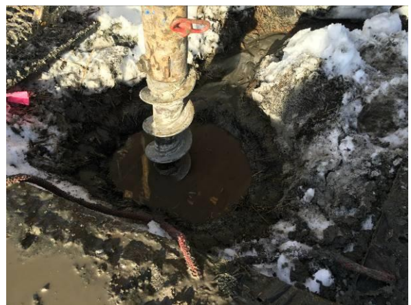
Photo #6 View at borehole 1358-9 (1) – groundwater stopped flowing at approximately 45 feet bgs.
