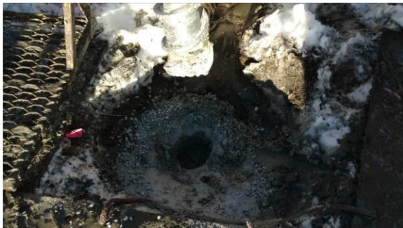
Photo #9 Sealing completion at borehole 1358-9 (3).
