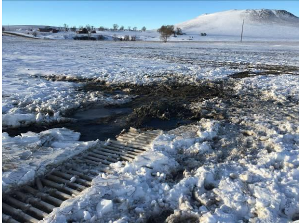
Photo #7 Sealing completion at borehole 1358-9 (1).
