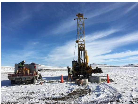
Photo #5 View east at the preparation of sealing borehole 1358-9 (1).
